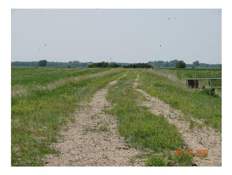
Photo 11: Monitor settlement of crest directly above the box culvert
