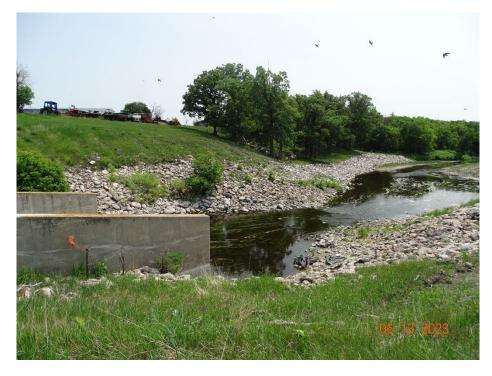
Photo 9: Riprapped downstream channel
