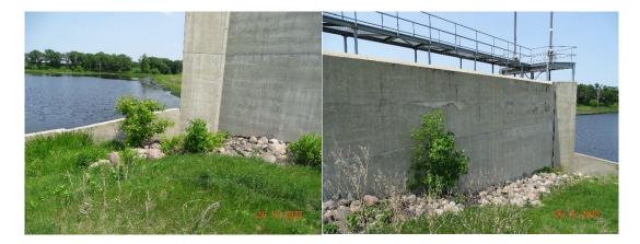
Photos 5 and 6: Trees and brush near concrete spillway to be removed
